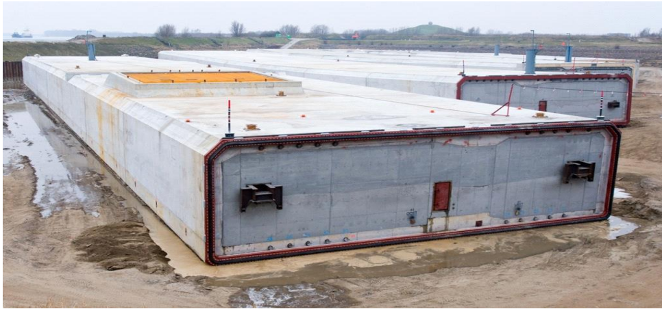
Figure 3. Segments of immersed tunnel ready 1
