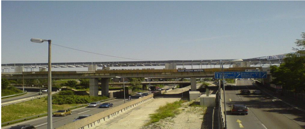
Figure 2. Entering in the tunnel under Danube in Vienna 1
